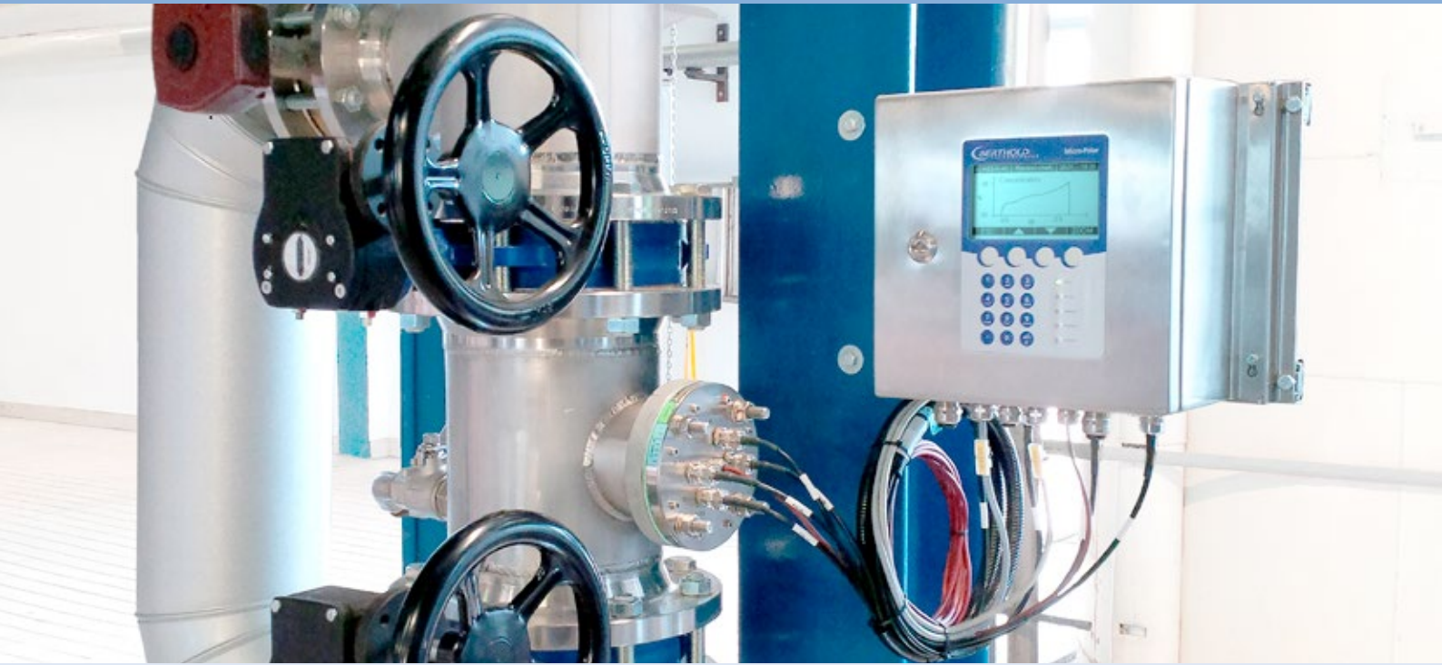
Determining the dry substance in a wastewater pipe – LB 566 with container probe installed in a pipeline.
